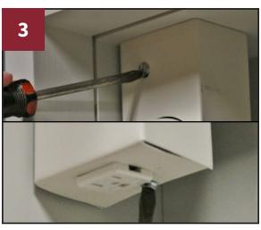
Unscrew electrical raceway
